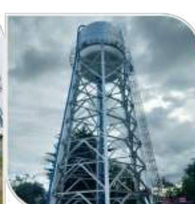
300 CU.M. ELEVATED STEEL TANK, CSWD COMPOUND, BRGY. FATIMA
