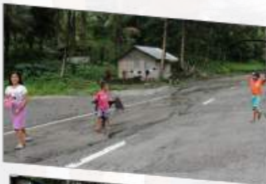
Taken before the pipes were donated. The residents had to walk long distance just to get water from the source.
