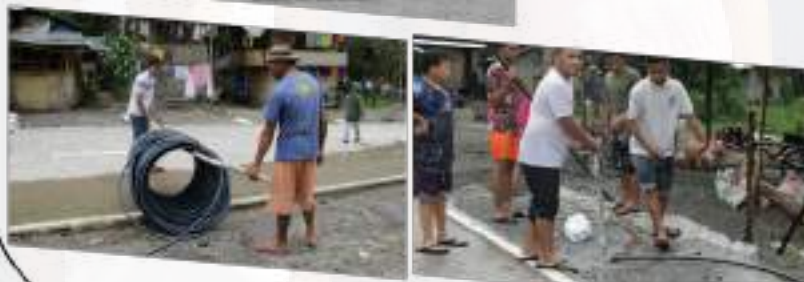
The residents of Sitio Tinefulan worked together to laid the pipes.
