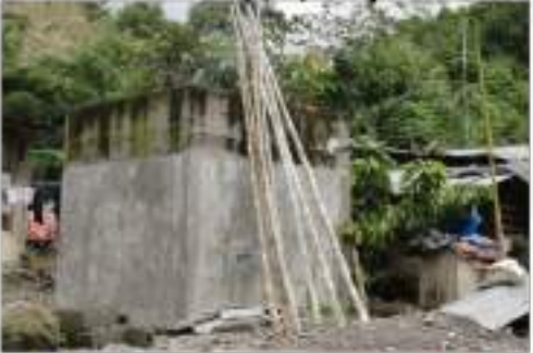
Water Tank (Before)
